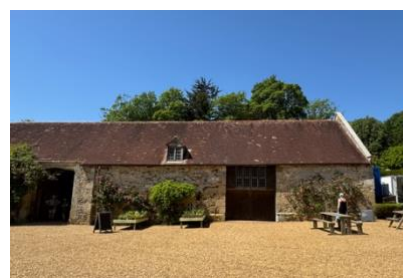
The Barn – the centre open area
